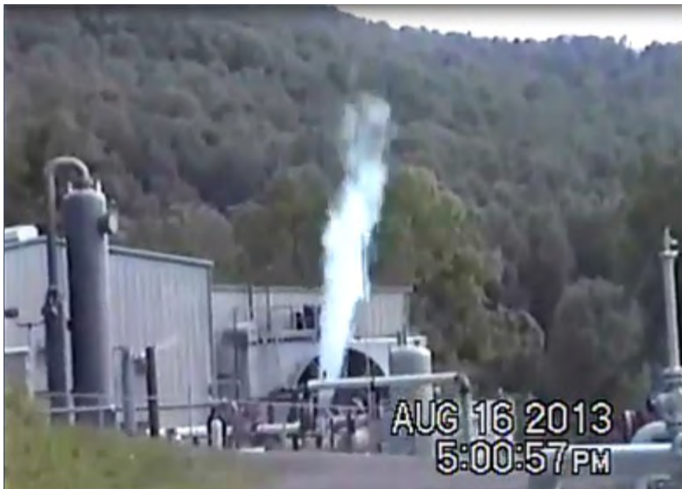
Figure 10. (a) Burnoff at Mark West processing plant, Houston, Pa. Photo courtesy of Bob Donnan. (b) Blowdown at Teel compressor station, Dimock, Pa. Video courtesy of Ron Teel.
